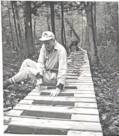
Shingling a boardwalk in the Maitland Woods
