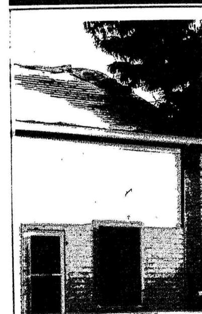
LIGHTNING left a large hole in the roof of this Chalk Street home, Saturday night. Averaged approximately 200 knots per hour. Normal winds at this time of year travel 100 to 120 knots per hour. McIlwraith photo.
